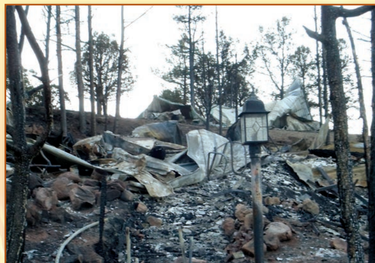
The Little Bear Fire destroyed this home and more than 250 other structures when it burned near Ruidoso in 2012. Photo courtesy of Kelly J. Hamilton, Southwest Border Food Protection and Emergency Preparedness Center.
