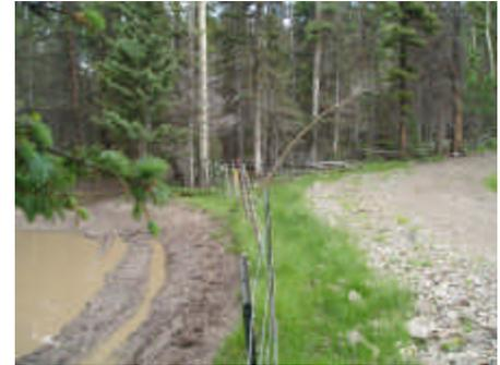
Left: Road improperly constructed and drained.
