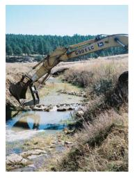
On the Sally Swift project a weir is being built with a track hoe from the stream terrace. Note the bank excavation on the left and then right below the track hoe arm.
