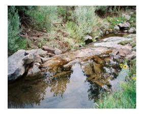
On the same property (at left), we took advantage of the bedrock to raise the streambed elevation some 10" by cementing two layers of rock to it. This structure, the only one of its type constructed there, was part of a series of structures installed throughout this incised channel reach.
