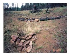
'02. On the Geney Nix property, 255' of logs were laid on contour to slow runoff down and assist with loss of soil and erosion.
