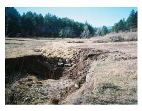
At the upper end of this work area were two more major head cuts one on each side of a earth tank berm. Several options were looked at and the one chosen was to rebuild the dam with an adequate spillway to accommodate a 25 year storm event.
