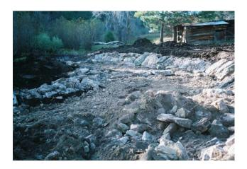
Boulders and rock for this spillway, the lower reconnection channel and the 9 structures involved, were harvested on site. This spillway required over 90yds<sup>3</sup> to complete. The above mentioned wetland area is in the photo's background.
