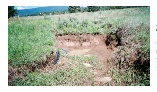
After a 30 minute, 2½" rain event in '06. This happened to two of the 4 log head-cut structures. One was rebuilt with adjustments to hopefully prevent this and the one pictured, will be re-done using boulders and rock.
