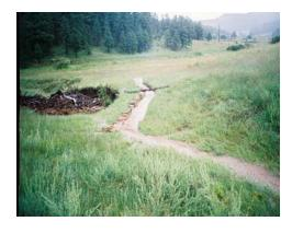
This last structure was built where we wanted to divert water again, from another arroyo (the logging road) on to flat land to help disperse the water more evenly. If we can break the single thread flow into numerous flows around the 40' edge of the lower outside rim of the half moon, the possibility of erosion is reduced completely.
