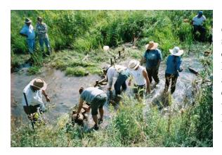
September, 05 induced meandering and stream bank stabilization work was completed on **3800**' of Manuelitas Creek. Most was done with heavy equipment, but a part was also completed with hand labor during an educational workshop held on the property. Picture to left, a cottonwood log vane being installed at Jones' property
