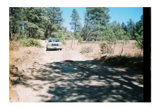
This work took about 6 hours using a track hoe to complete as we moved the machine down to do our planned stream restoration work. It was the first time this contractor built a rolling dip and he caught on to the design and concept after doing the first one. Fixing the road and reducing sediment loading to Arroyo Horno's stream were two objectives, along with using it for a future demonstration site.
