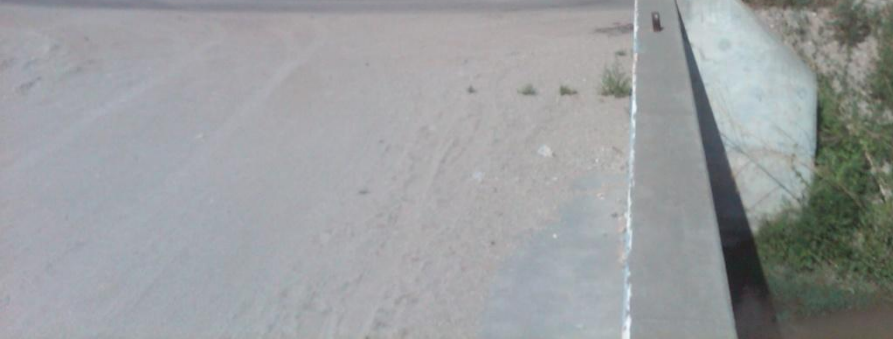
Flood Control Apron
